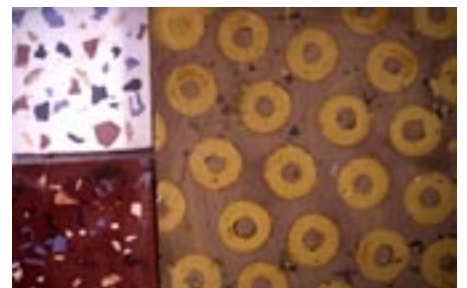
Coloured plaster marquetry. A surface depression, made by a mould is filled with plaster of another colour. Plaster 'terrazzo' and a pattern suggested by 'potato stamps'
