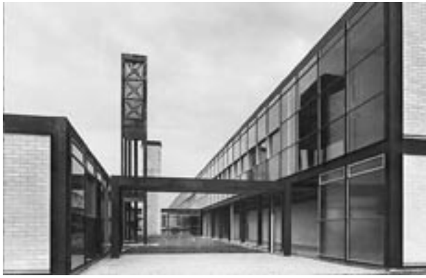
Hunstanton school, in Norfolk, won by Alison and Peter Smithson fresh from college, enflashed 18C 'Illuminismo' ideas of transparency and constructive clarity. Its environmental defects ensured the Smithsons had no Public jobs for 25 years - until the disastrous Robin Hood Gardens.
